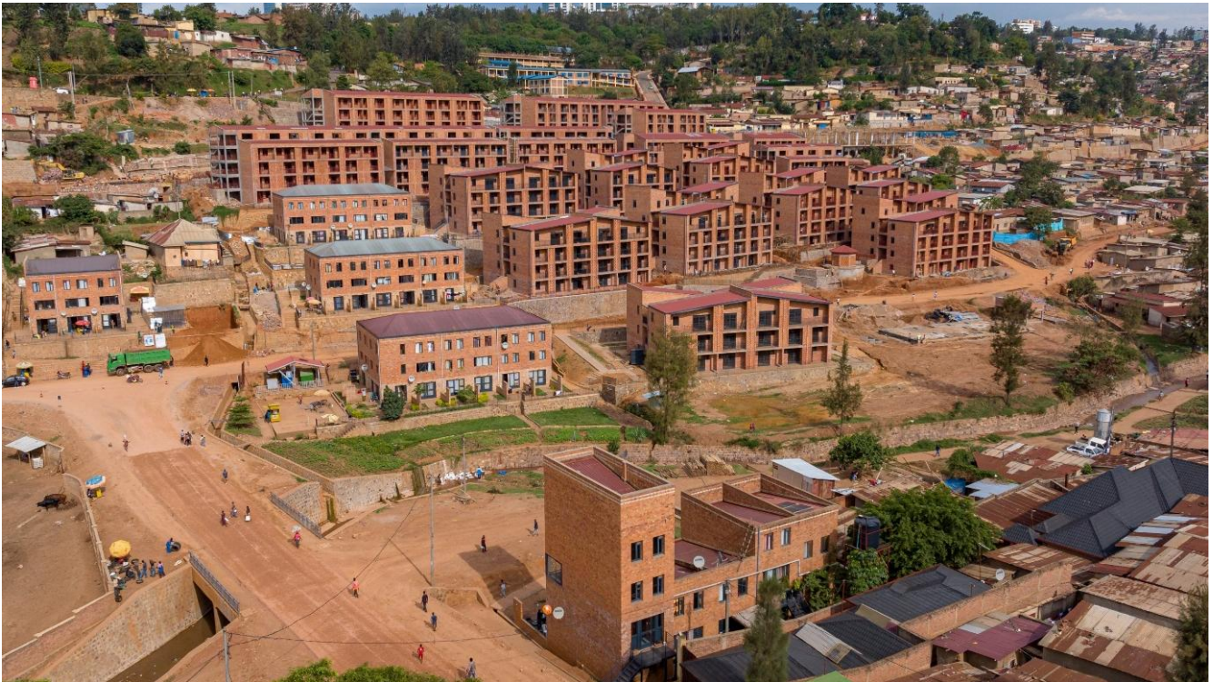
Mpazi construction progress, February 2025. City of Kigali.
