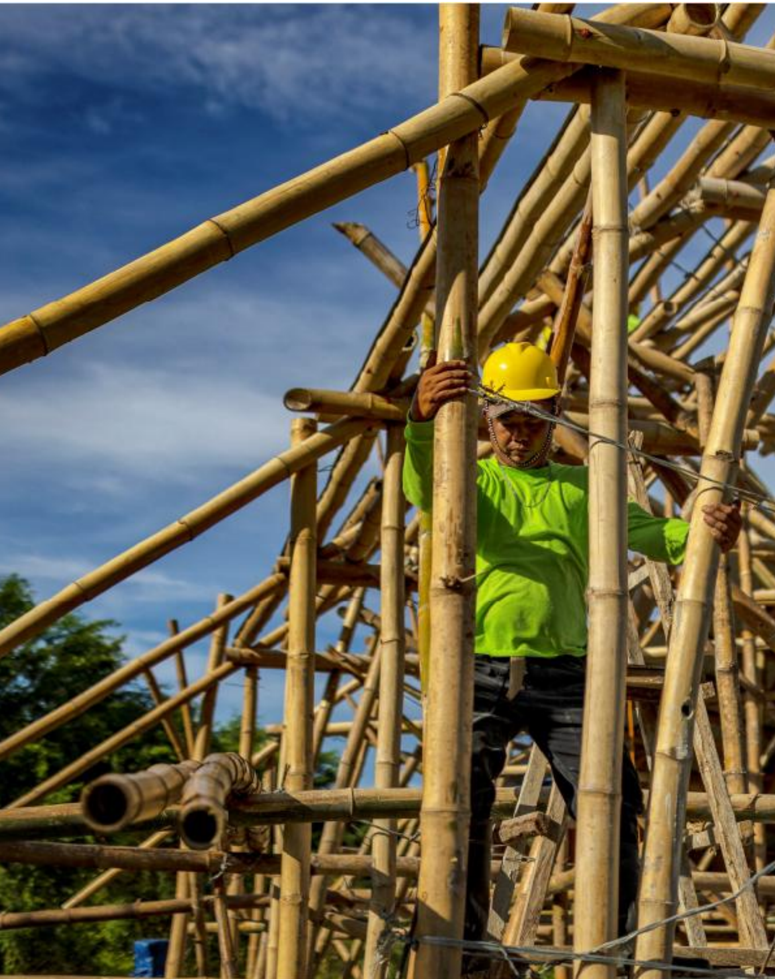
Bamboo building frame, Philippines. Hilti Foundation and Base Bahay Foundation Inc.
