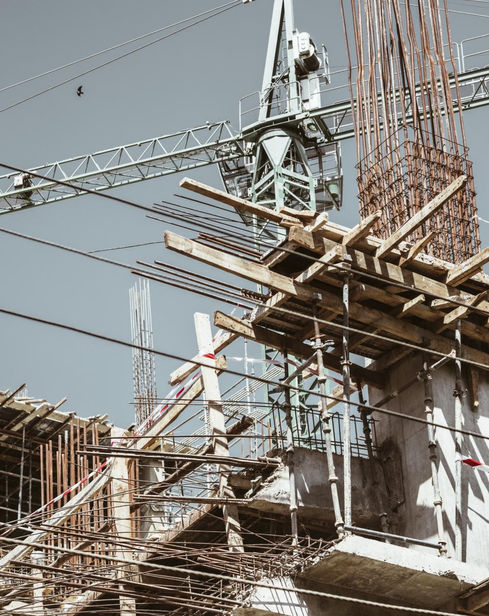
Concrete construction, Kenya. Nirian/iStock
