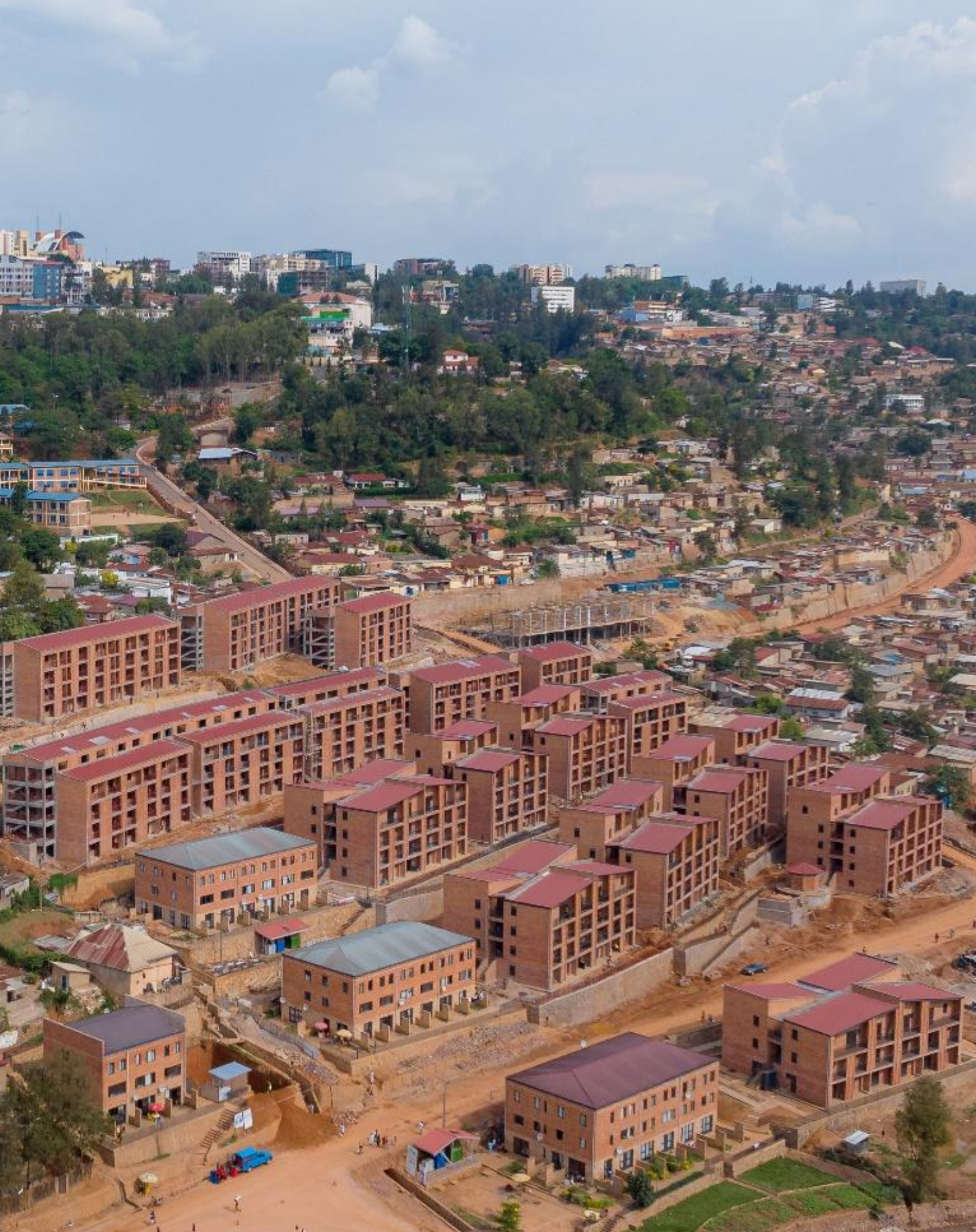
Mpazi redevelopment, Kigali, Rwanda: City of Kigali
