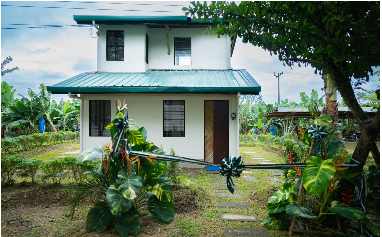
Two-storey bamboo prototype. Hilti Foundation and Base Bahay Foundation Inc.
