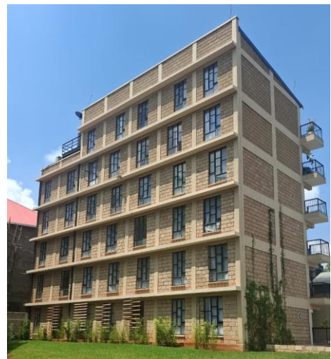
Figure 1 : ZIMA Courtyard in use by community
